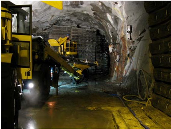
Grouting tests in Äspö HRL
